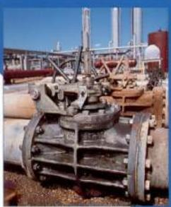
Grease, oil, dirt, surface corrusion, and failing paint were removed from equipment inside and outside this petrochemical plant, without the shut-down of adjacent equipment.
